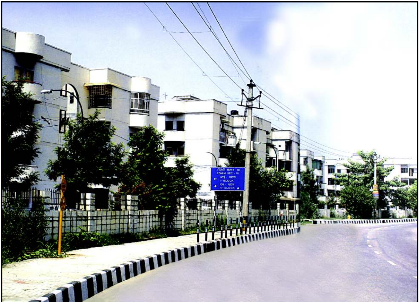
Pic. A curvilinear view of DDA apartments in Rohini
